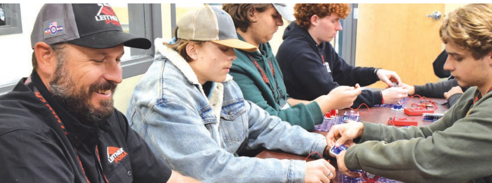
Tim Brosnan, eastern general manager at Leitner-Poma of America, works with students on electrical panels, showcasing some of what it takes to become a lift mechanic
